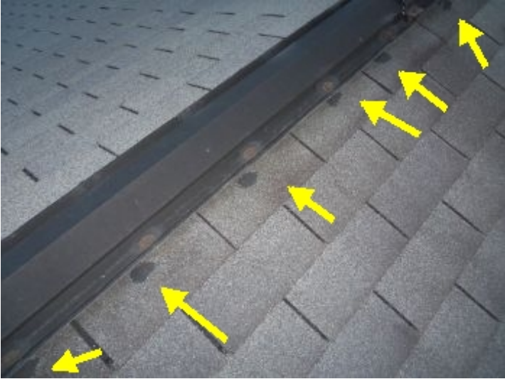
exposed fasteners
