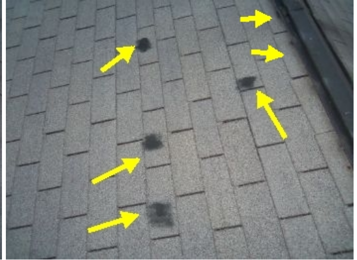
exposed fasteners
