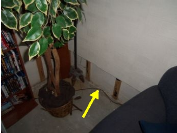
removed drywall from basement wall
