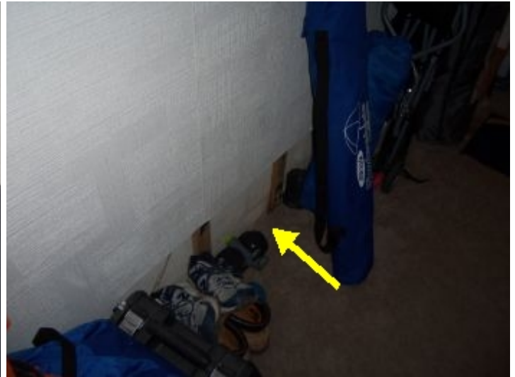
removed drywall from basement wall
